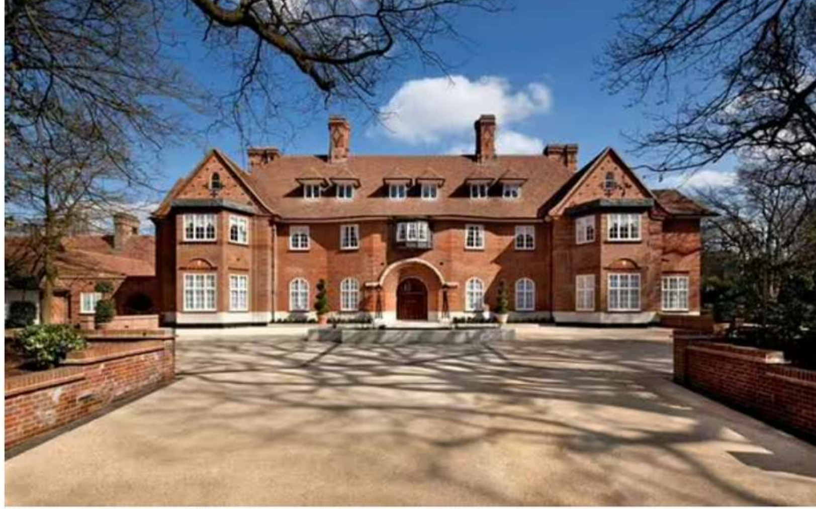
Heath Hall was bought as a wreck in 2005 before being refurbished and put back on sale for £100m (Image: SWNS.com)
