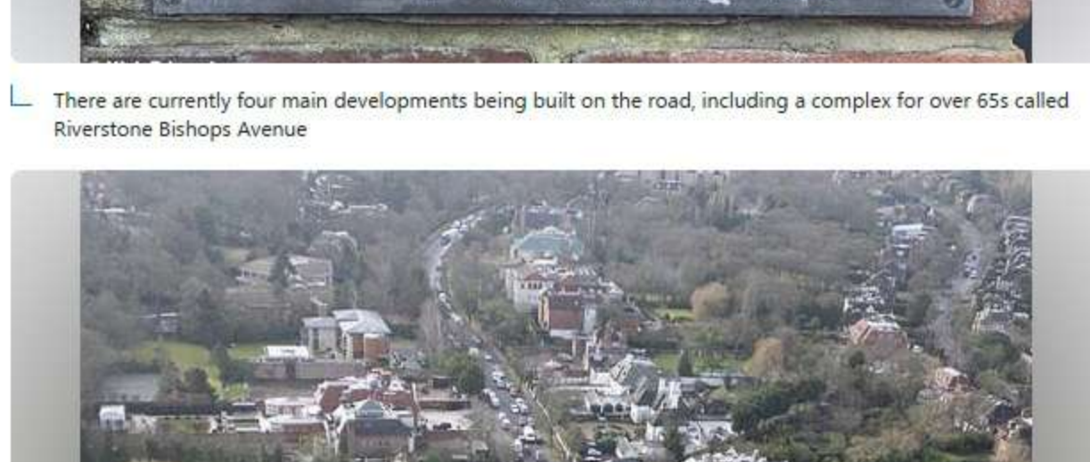
There are currently four main developments being built on the road, including a complex for over 65s called Riverstone Bishops Avenue
