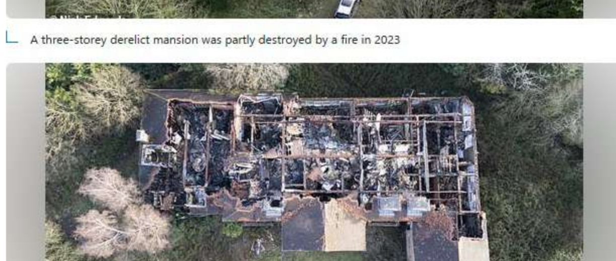
A three-storey derelict mansion was partly destroyed by a fire in 2023
